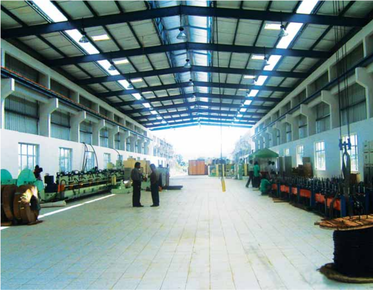
New doorframe plant coming up at Pune
